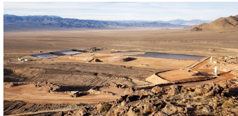
Overlooking Heap Leach & Process Facilities
